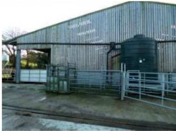
Gravity above ground storage with filter unit at top left (courtesy of ADAS)
