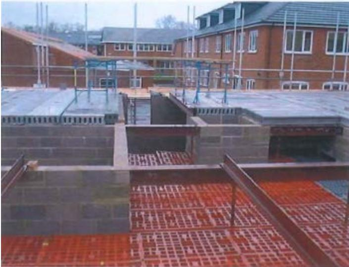
'Typical PDS used in a domestic housing construction setting (courtesy of *Tarmac*)'.
